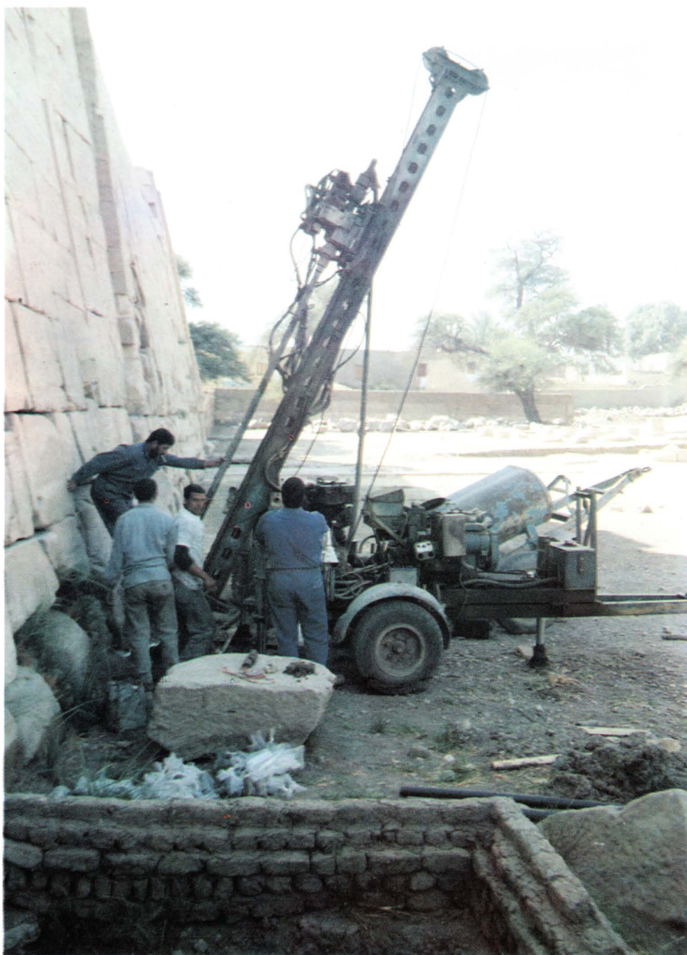
Inclined coring in the pylon foundation. [Cliché Hany Helal].
